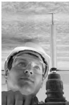
EZE220 drive sleeve slips over drill bits to ease installation of HangerMate® anchors in concrete.
