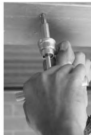
EZE290 tool speeds installation of HangerMate® LG anchors.
